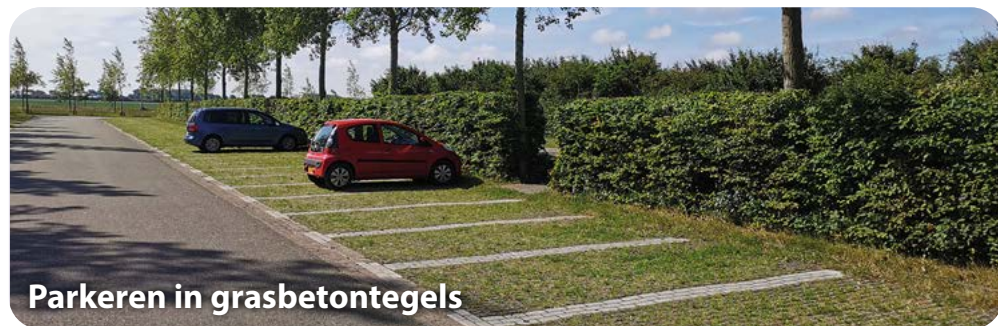
Parkeren in grasbetontegels
